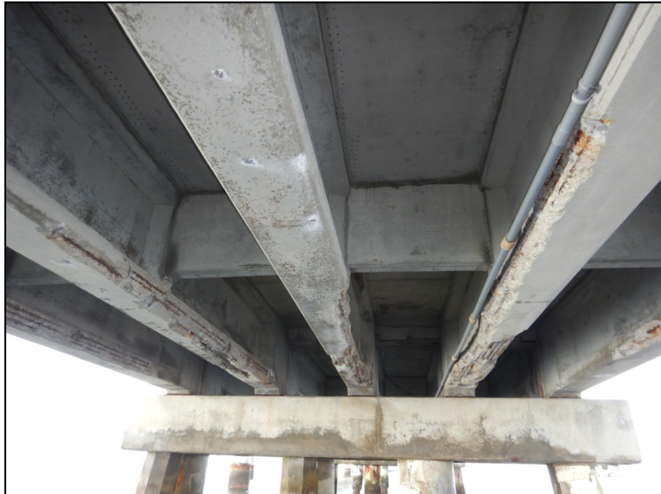
Photograph 4: Prestressed Girder Arrangement - Spans 1 through 18
