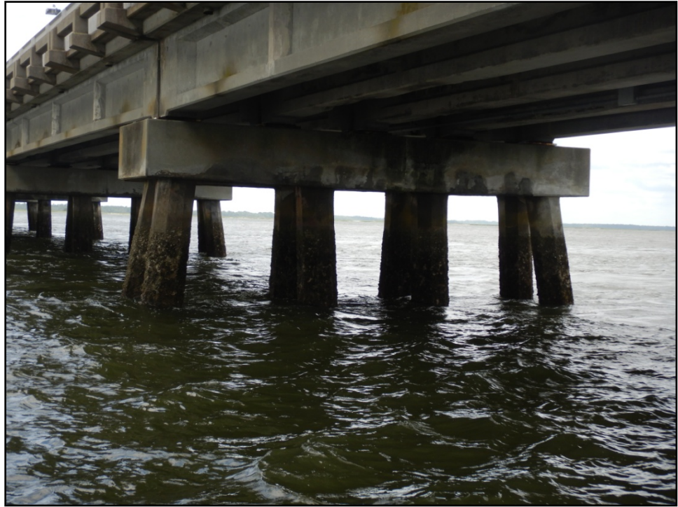
Photograph 1: Typical 8 Pile Bent
