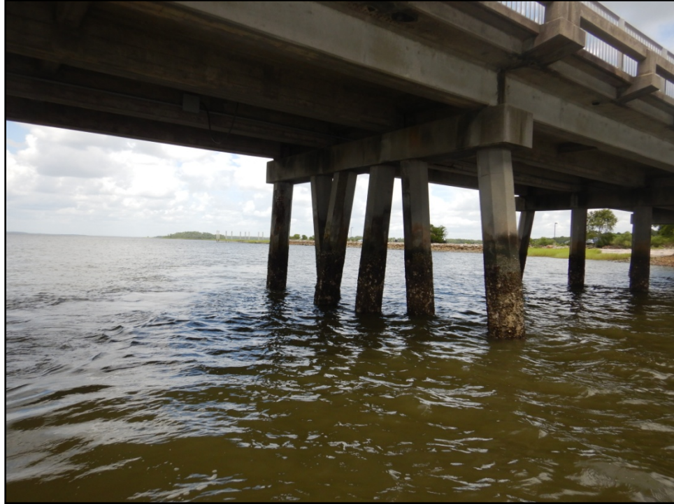
Photograph 3: Typical 6 Pile Bent
