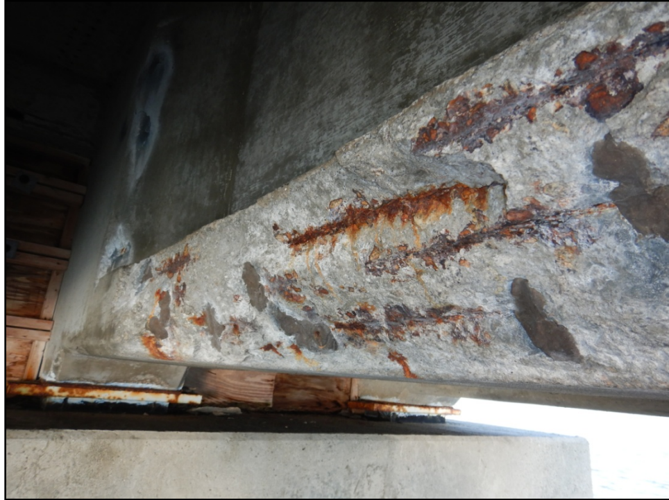
Photograph 5: Typical Prestressed Concrete Girder Repair
