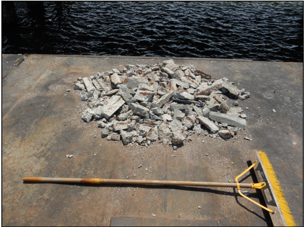
Photograph 12: Deteriorated Concrete Removed from Spans 19 through 29
