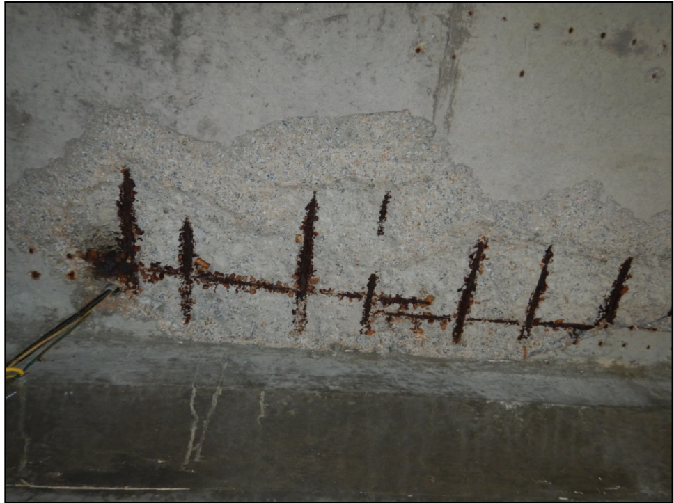
Photograph 9: Underdeck Spall
