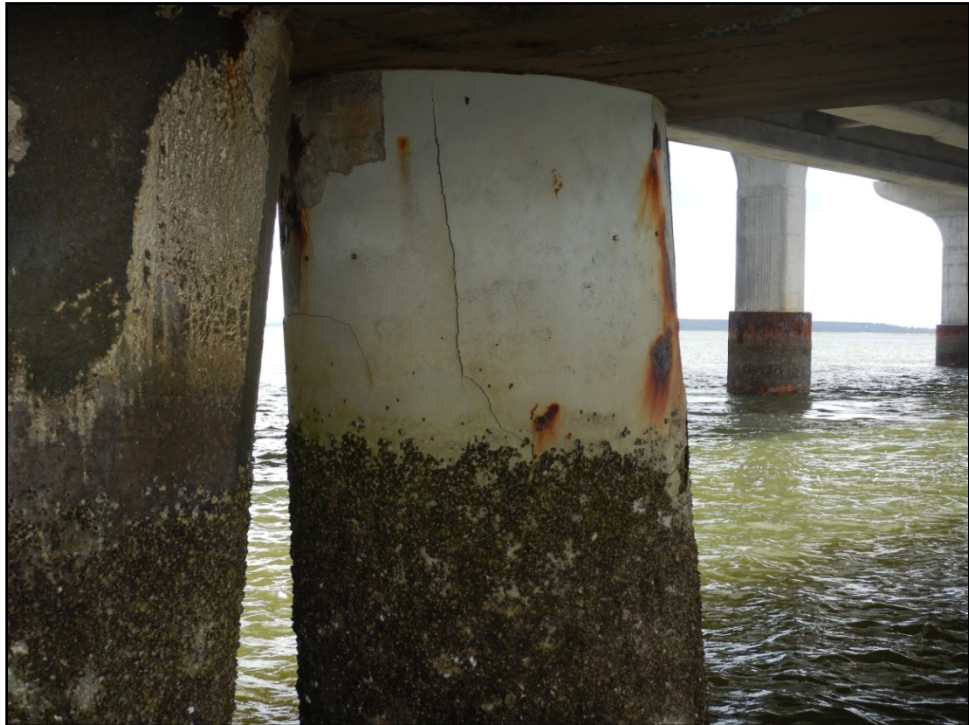
Photograph 14: Typical Pile Condition Above the Waterline
