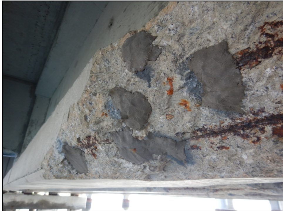
Photograph 6: Typical Prestressed Concrete Girder Repair
