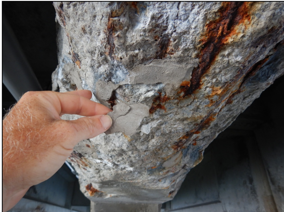
Photograph 8: Prestressed Concrete Girder Repair with Minor Delamination
