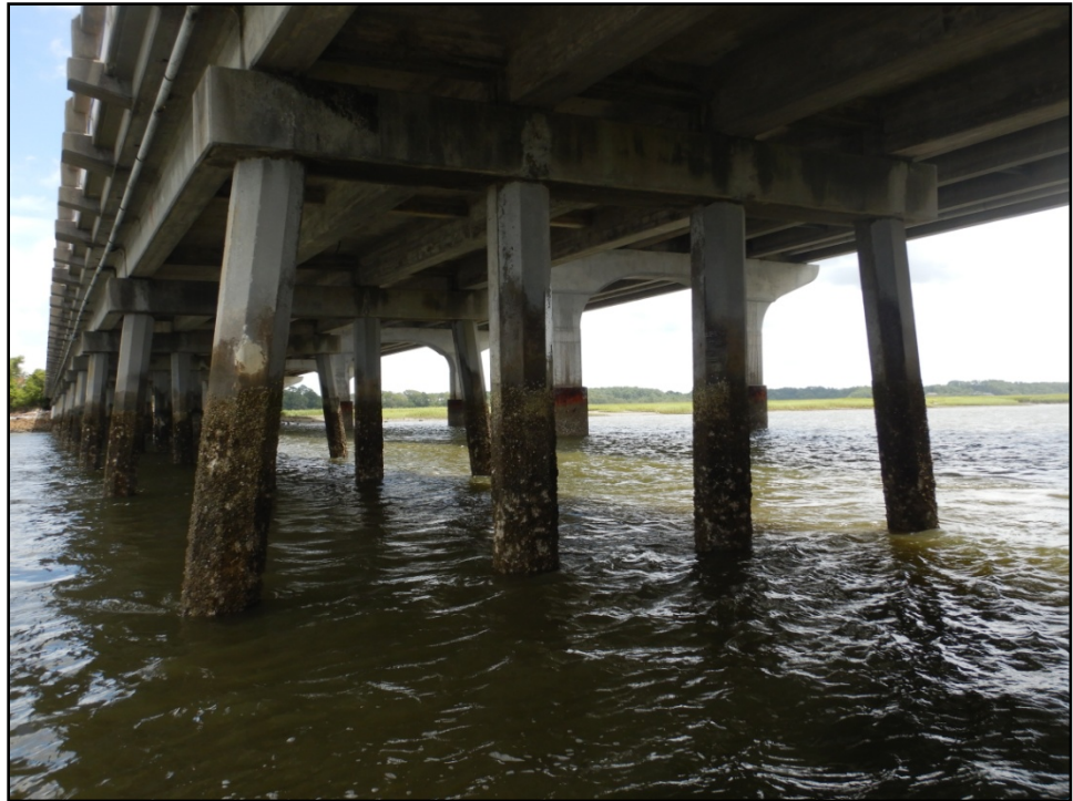
Photograph 2: Typical 4 Pile Bent
